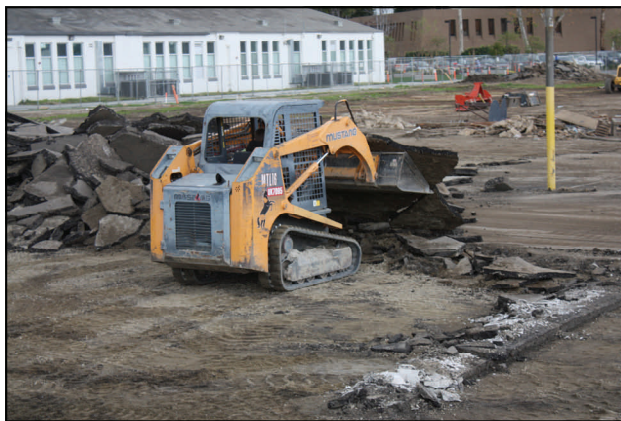
Tearing Up the Field — A small tractor rips up asphalt as part of the effort to prepare the area for its new grass.
